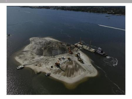
Nearly all the fill required to complete the north island has been delivered to the site. Over the next couple of months, crews will finalize the island's shape, compact the fill to achieve the correct intertidal elevations and then place limestone rocks along its outer rim.
